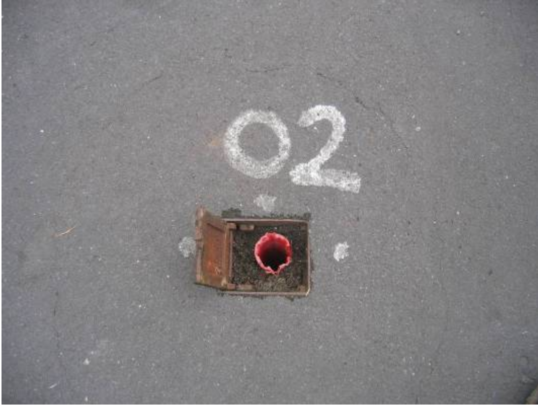
Plate 21 Scarborough South Cliff H4 (AA02)
