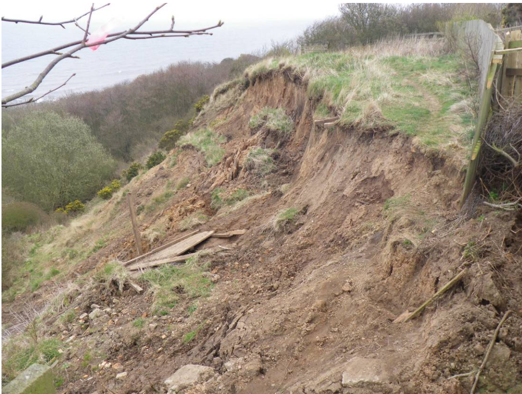
Plate 4 Slope failures on Cornelian Bay side looking east (14 th April 2010)
