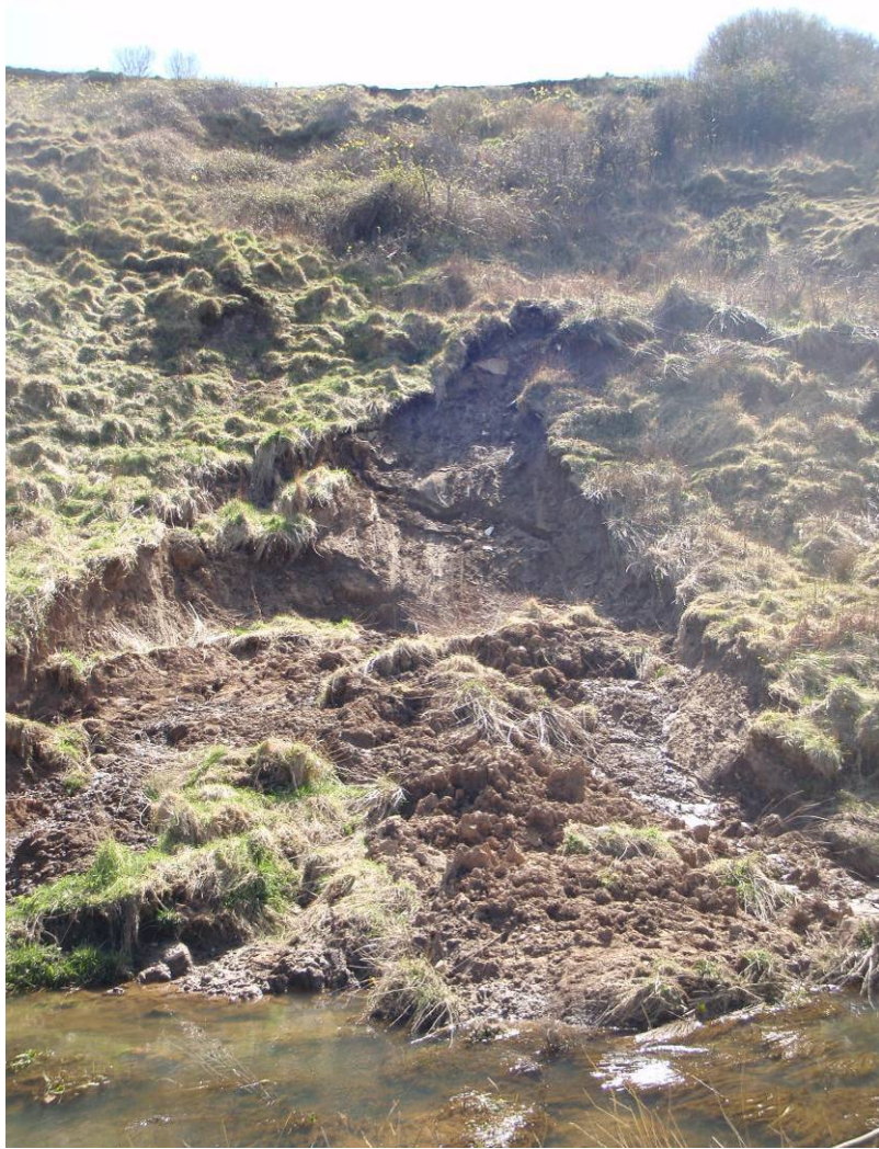
Plate 4 Slope failure along river's edge of Behavioural Unit I. (14 th April 2010)
