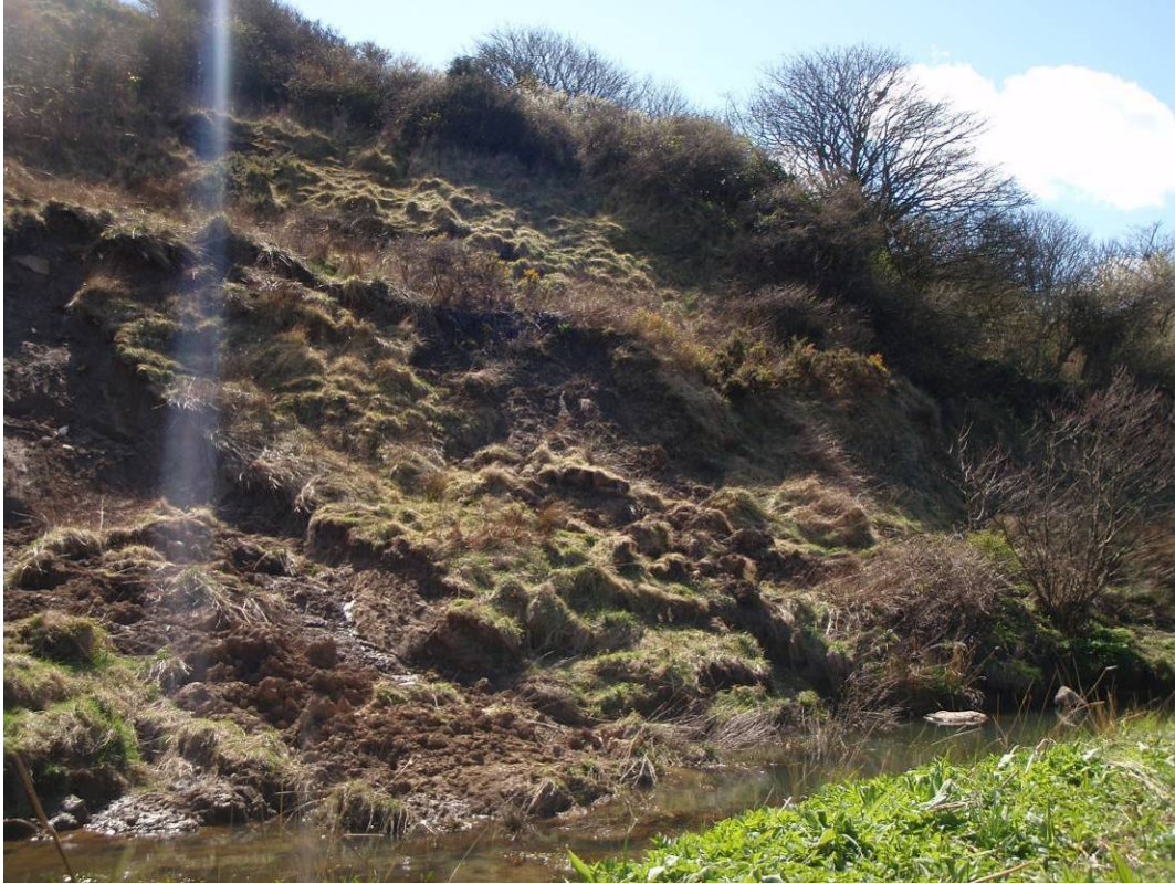
Plate 5 Slope failure along river's edge of Behavioural Unit I. (14 th April 2010)
