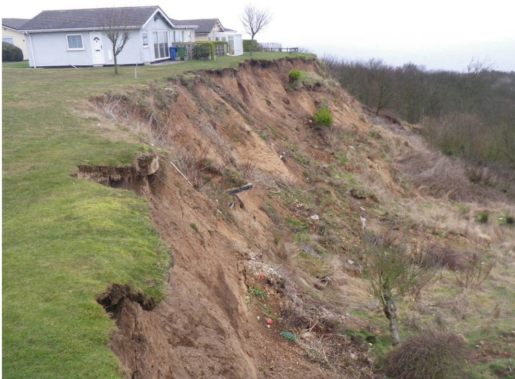
Plate 11 Cliff recession at Knipe Point Headscarp (8 th March 2010) looking east
