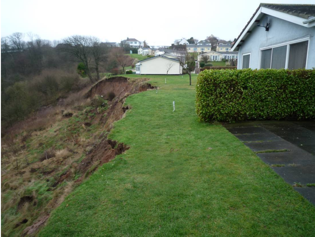
Plate 7 Cliff recession at Knipe Point Headscarp (20 th January 2010)
