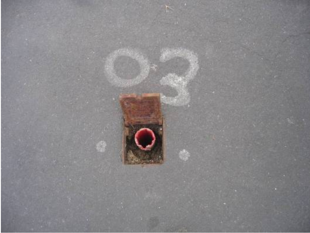
Plate 23 Scarborough South Cliff H6 (AA03)
