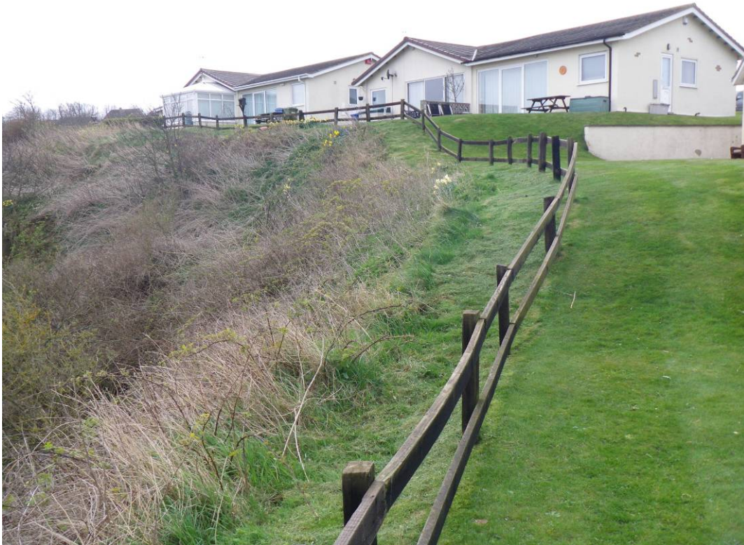
Plate 5 View of Knipe Point Headscarp at Monitoring Pin H4 (14 th April 2010)
