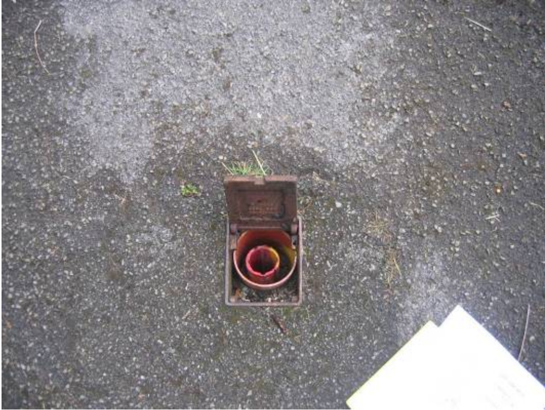
Plate 29 Scarborough South Cliff D3 (AA08)
