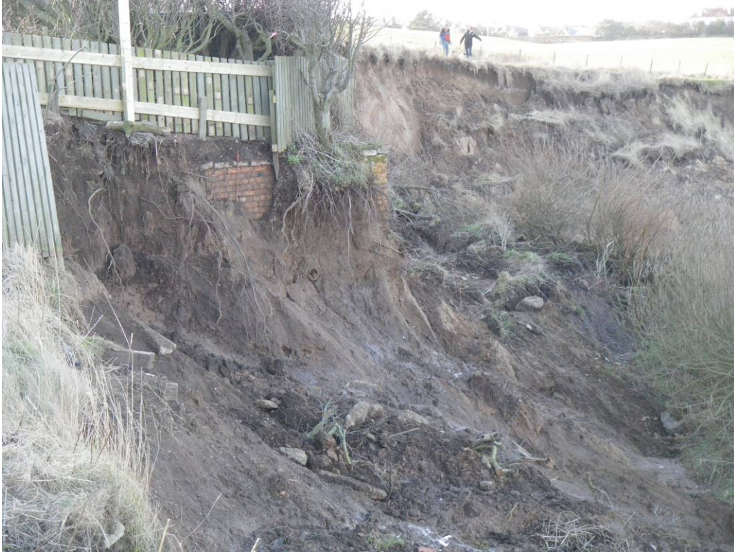
Plate 1 Slope failures on Cornelian Bay side of Knipe Point looking northwest
