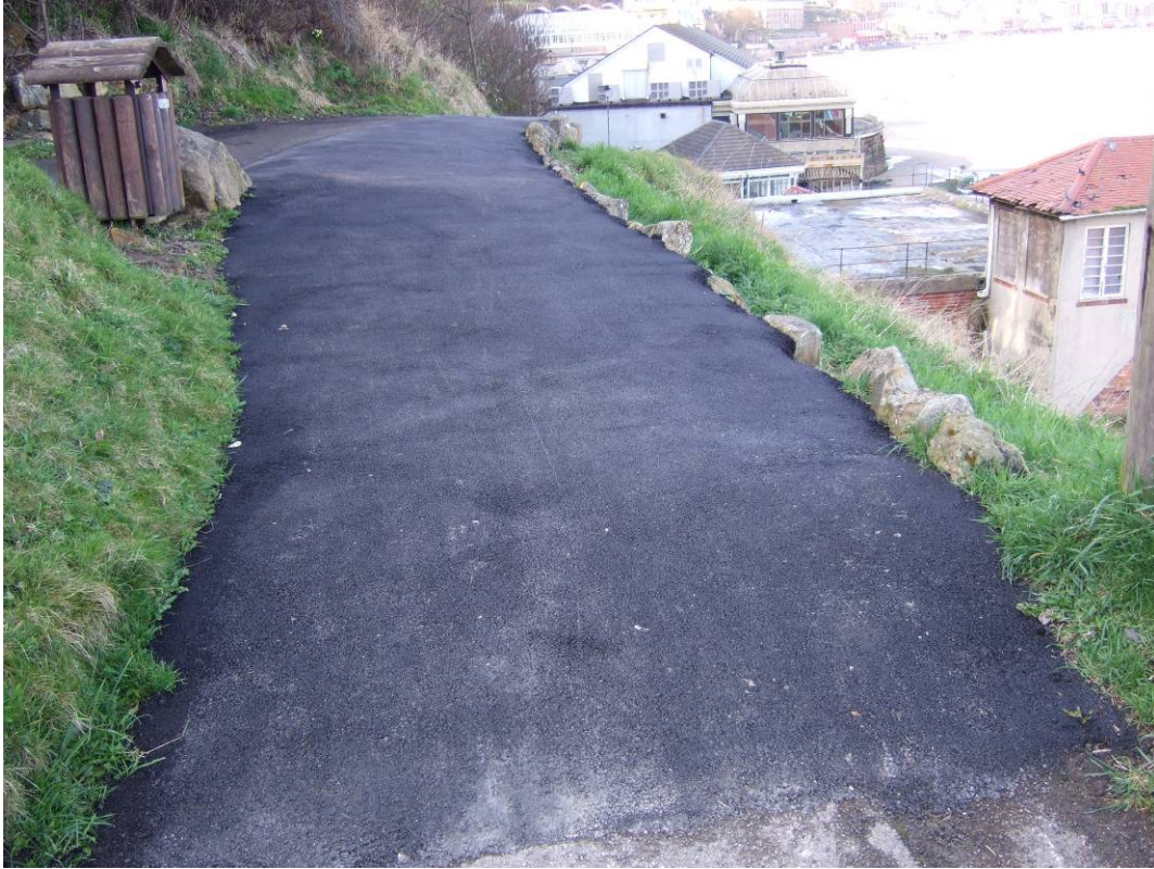
Plate 55 Scarborough South Cliff. Pavement repair above the Clock Café (April 2010).
